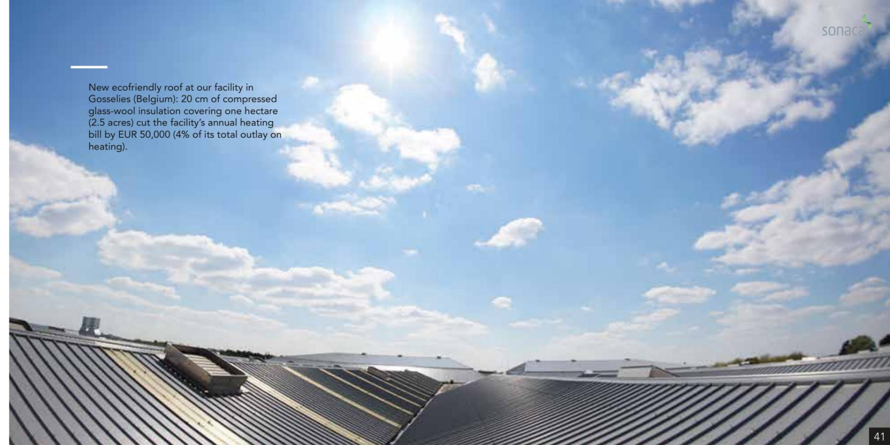
New ecofriendly roof at our facility in Gosselies (Belgium): 20 cm of compressed glass-wool insulation covering one hectare (2.5 acres) cut the facility's annual heating bill by EUR 50,000 (4% of its total outlay on heating).
